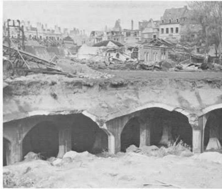
FIGURE 61.—Bombed-out underground reservoir at Cologne, Germany, which normally stored more than 5 million gallons of water.
